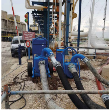
J4"D Station d'épuration.
