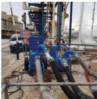
J4"D Station d'épuration.
